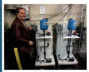
It turns out that zapping salt water with low-voltage electricity creates a couple of powerful yet nontoxic cleaning agents. Sodium ions are converted into sodium hydroxide, an alkaline liquid that cleans and degreases like detergent, but without the scrubbing bubbles. Chloride ions become hypochlorous acid, a potent disinfectant known as acid water.
